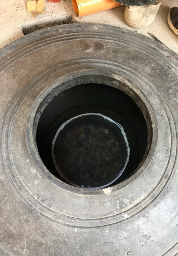
Inside STP Tank
